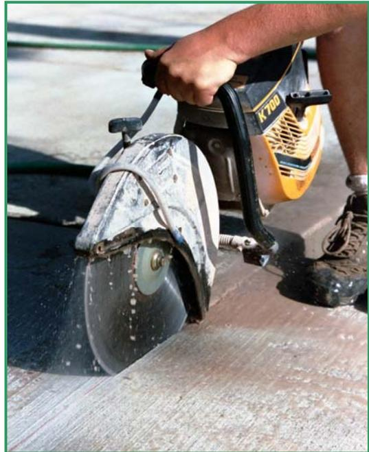
Photo showing cutting of control joint
