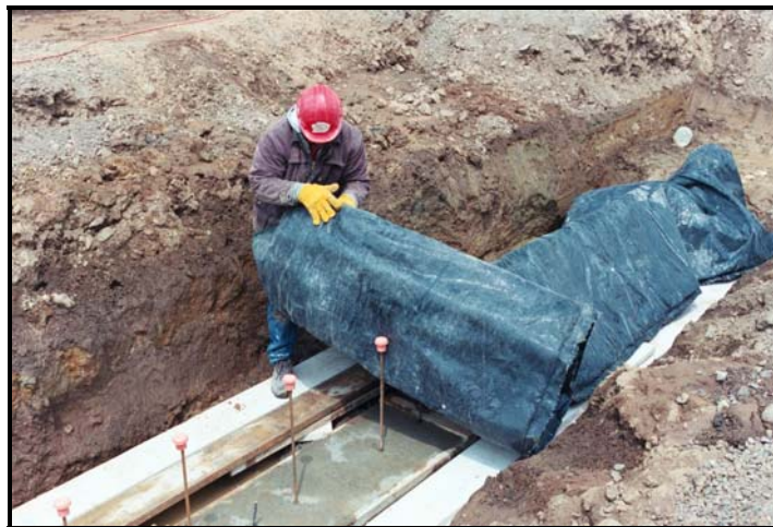
Protection of concrete using insulating blanket
