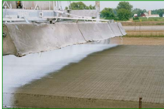
The use of plastic, fog sprayers, and/or evaporation reducers along with proper curing (shown above) are essential
